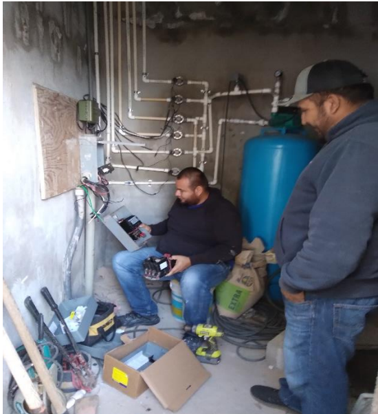
Backup Pump Circuit Breaker Installation
