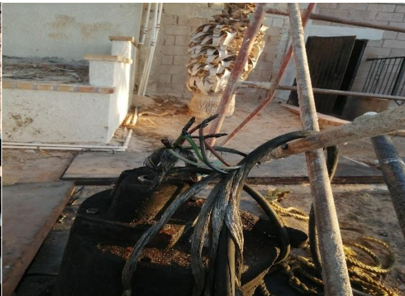
Backup Sewer pump Auto Cutover Test
