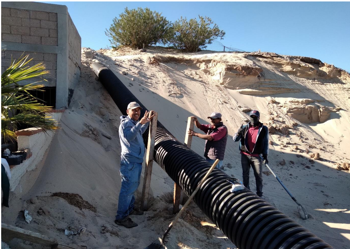
Laying of New Drainage Pipe.
