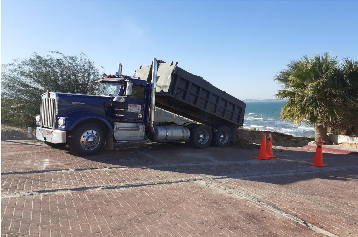
Backfill of ravine.
