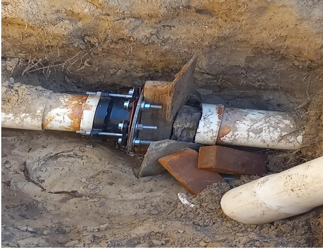
Temp repair to return water service to La Hacienda
